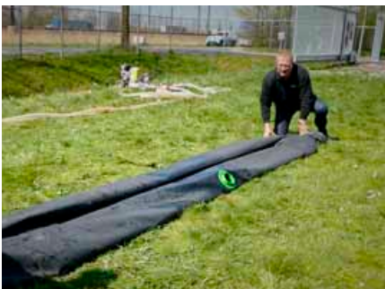
Then fold the SLAMDAM® back half.
