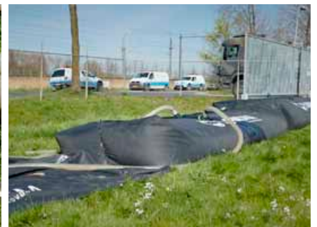
Start pumping to remove the water.
