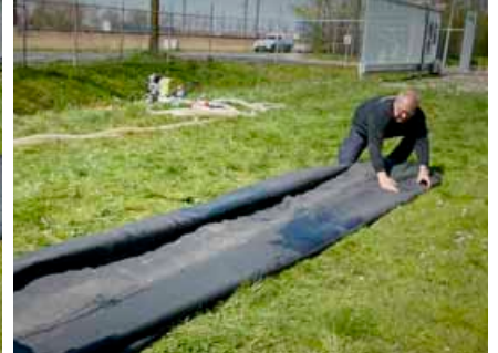
Also fold back a quarter of the SLAMDAM® on the right side.
