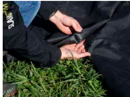
Place the one SLAMDAM® 2 cm over the other for good closure and watertightness.
