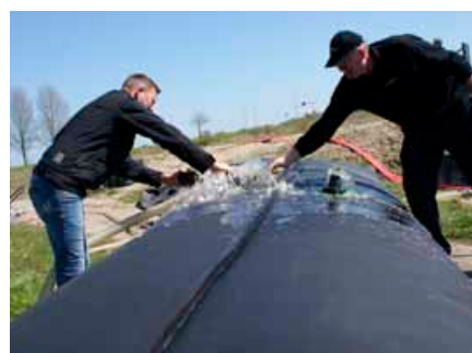
While disconnecting the hose, let some air escape.
