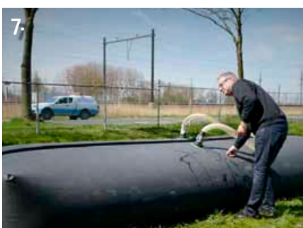
7. Fill the SLAMDAM® to a height of about 67 cm.
