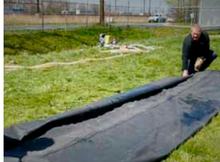
Fold back a quarter of the SLAMDAM® on the left side.
