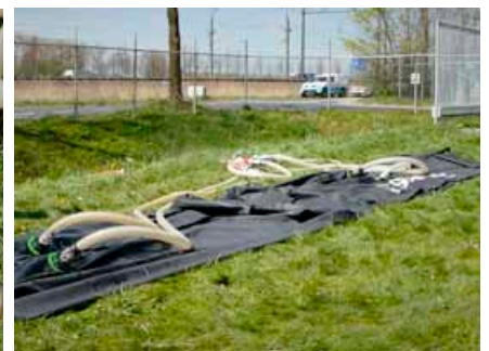
The SLAMDAM® is now ready to be filled with water. Both SLAMDAM® compartments must be filled simultaneously.
