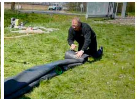
Roll in accurately from both sides towards the filling points.
