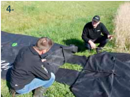
4. Place the next empty SLAMDAM® and follow the line of the first SLAMDAM®.
