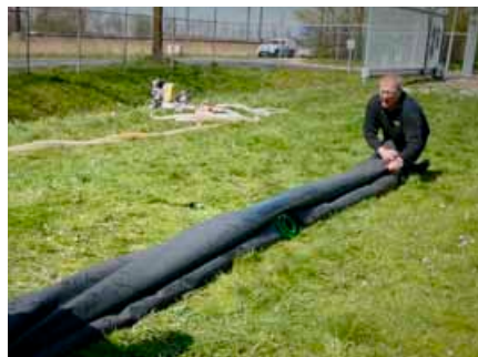
Make sure the filler caps remain free, so as much water as possible will be removed.
