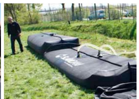
By repeating this steps, length is created by placing several SLAMDAMS in a row like a chain.
